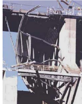
Fig. 6 Folsom dam (1995), gate failure [Vogel, 2014]
