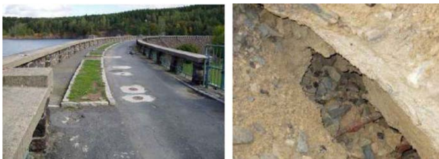
Fig. 9 Mostiště (2004), piping through dam core [photo VD - TBD a.s.]
