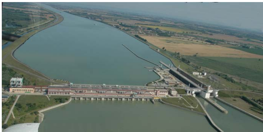
Fig. 2 Hydraulic Structure Gabčíkovo
