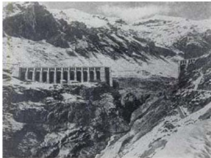
Fig. 2 Gleno dam(1923), collapse of dam block [Herzog, 1999]
