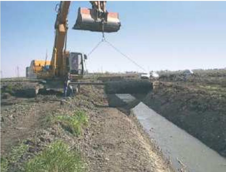
Fig. 5 Installation of beaver netting along Canale Zabarelle
