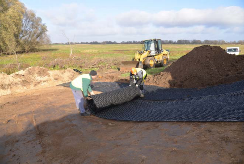
Fig. 4 Installation of beaver netting
