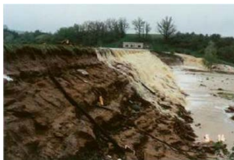
Fig. 8 Pocheň (1997), overtopping and surface erosion [photo: Žatecký 1997]
