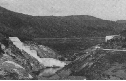
Fig. 3 Malpasset Dam(1959), foundation failure [Duffaut, 2013]
