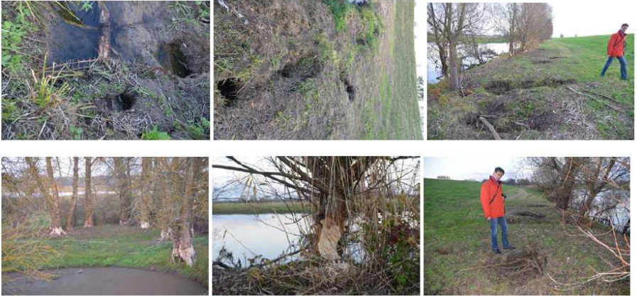
Fig. 3 Effects of beavers in floodway encroachment zones
