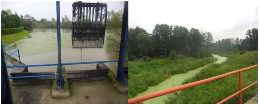
Fig. 3. Eutrophication and sedimentation caused by the “Syphon” (left) and Eutrophication impact in Stream Želin (right)
