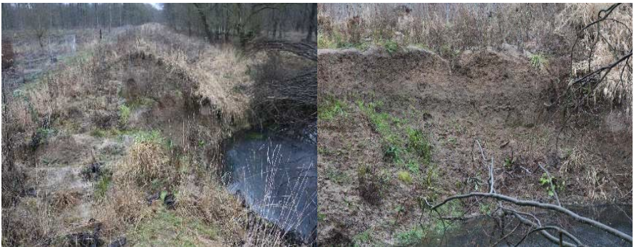
Fig. 3 Typical breach appearance (left) at quasi-homogeneous levees (“old” levees) with distinctive stratification of the levee body (right)
