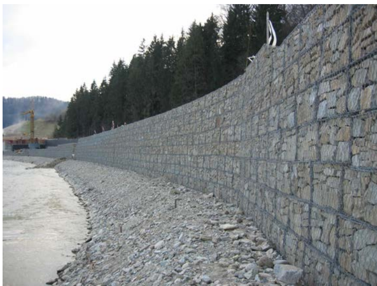
Fig. 4 Gabion river wall at Oravský Podzámok, Slovakia
