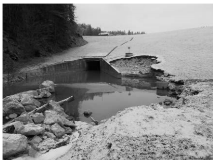
Fig. 3 The scour hole on the left side of the stilling basin prior to refurbishment works
