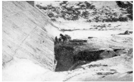
Fig. 4 Ashley Brook Dam (1909), foundation failure [Vogel, 2013]
